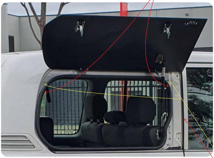
Snug up all the previously loose bolts whilst aligning the window. Pay attention to how level it is across the base and the way the door seal interacts with the window edge.
